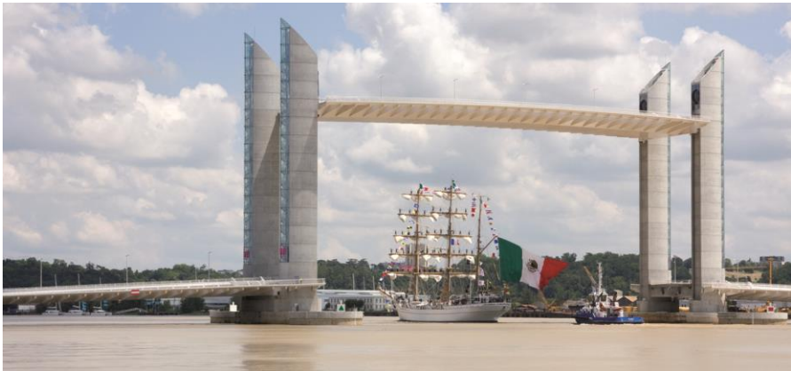
The bridge Jacques Chaban-Delmas , inaugurated in March, 2013 in Bordeaux
